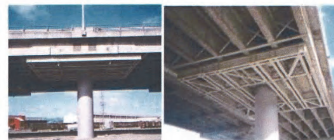
Figure 2.3. Column piers either side of where the Wellington Fault cuts the line of the Thorndon Overbridge have retrofitted "catch frames" with the capacity to accommodate lateral fault displacement of the order of 4-5 m between piers and prevent span collapse in the event of surface rupture of the fault. Photos: Billings, I.J. and Powell, A.J. (1996).
